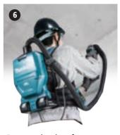
Prevent the dust from scattering by using dust extractors on the grinders to protect operators from respiratory diseases DRILLING
